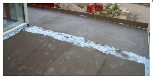
Installers used PCI Seccoral 2K Rapid fast-setting special waterproofing slurry to seal the upper side of the insulation panels. The fastsetting special waterproofing slurry prevents water ingress into the space below the terrace - this is a given.
