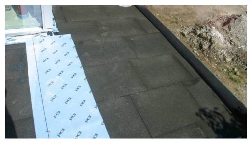
Terrace and flat roof in one: a garage is located under the terrace of the Murnau property. Mineral glass foam panels fixed in place with PCI Pecimor DK bitumen adhesive therefore insulate the space against the cold and protect the upper covering against water vapour.
