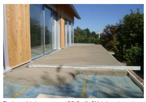
The layer of drainage mats and PCI Pavifix DM drain and screed mortar acts like a support layer. The mat and mortar system ensures fast and immediate drainage.
