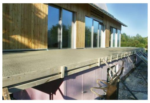
The substrate is now ready for the tiles to be laid. A drainage system ensures that rain and storms present no risk to the subsequent layer of porcelain stoneware. Under the drainage, a system comprising a bituminous layer, insulating panels and a waterproofing slurry safety layer ensure the garage located under the terrace remains dry.
