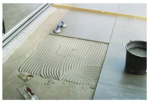
The installers used PCI Rapidflott fast-acting flowable mortar in conjunction with PCI Lastoflex polymer modified additive to cement the new 90 cm x 90 cm porcelain stoneware tiles to the Murnau terrace. The product mix is water-, frost- and weather-resistant, and therefore ideal for laying ceramics outside.
