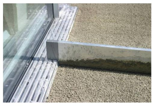
Exactly at the right height: the floor-to-ceiling windows which separate the living space from the terrace presented a special challenge. To prevent the new porcelain stoneware tiles creating a trip hazard, the construction professionals worked according to precise dimensions.
