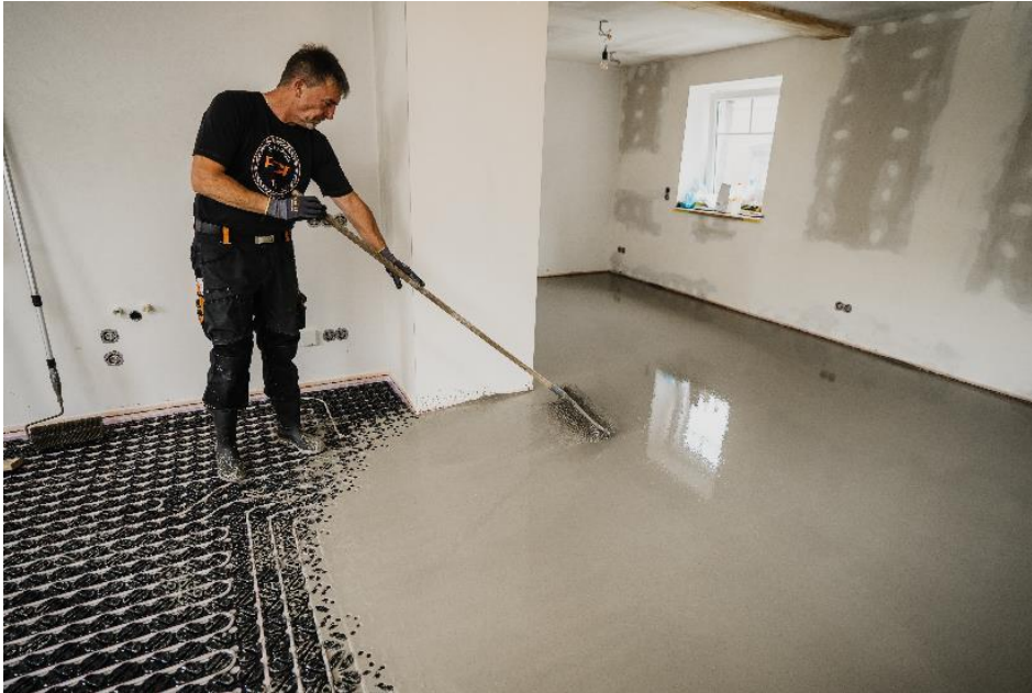
PCI Periplan Extra is self-leveling and therefore easy to work with. (© PCI Augsburg GmbH, Link to high-resolution photo)
