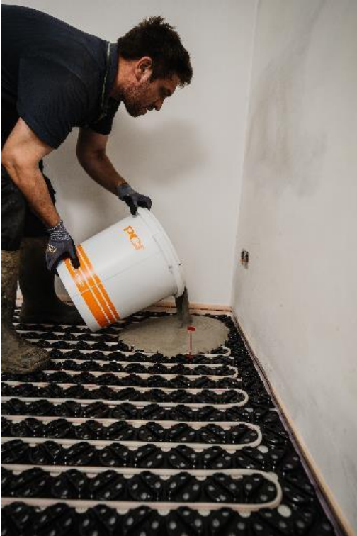
XPS insulation boards bonded with PCI Barraseal Turbo followed by the thin-layer underfloor heating only 17 mm high. (© PCI Augsburg GmbH, Link to high-resolution photo)
