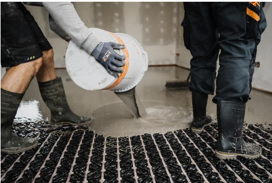
Roth's ClimaComfort® Compact system was cast with the fiber-reinforced special filler compound PCI Periplan Extra. (© PCI Augsburg GmbH, Link to high-resolution photo)
