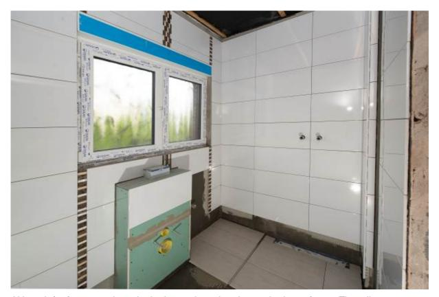
Although far from complete, the bathroom has already acquired new forms. The toilet now stands where the bath used to block access to the rest of the room. Standing in the space previously occupied by the toilet, and therefore much more accessible, is a floor-level shower.
