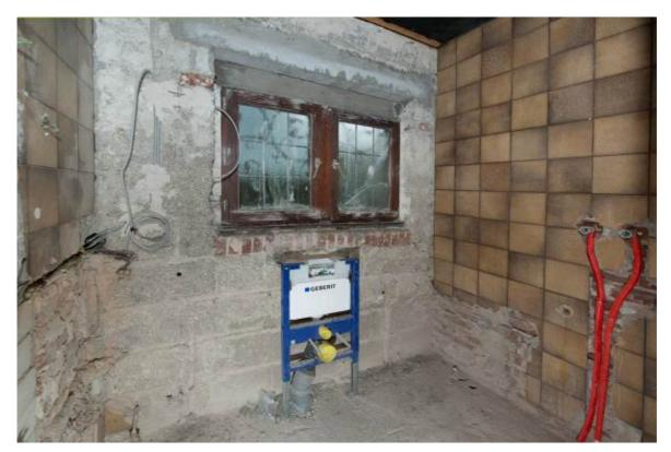
Out with the old: giving the small bathroom a new look and contemporary features entailed removing the floor tiles and some of the wall tiles. The installation of the bathroom fittings, which formed the preparatory work, was carried out by Gilbert Karwatzki from Essen.
