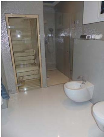
Fig. 3 and 4: The tilers covered about 40 m<sup>2</sup> of walls in the bathroom with 33 x 100 cm wall tiles.
