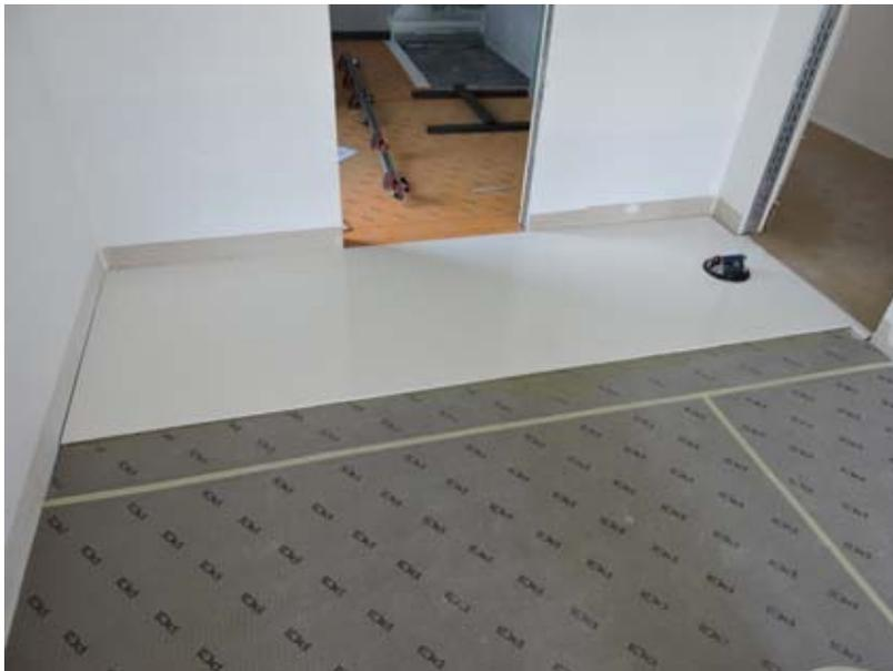
Fig. 7: To absorb stresses, the tilers installed PCI Pecilastic E insulating membrane with PCI Flexmörtel S1 Flott flexible adhesive under the tiling. The insulating and waterproofing membrane PCI Pecilastic U was used in the bathroom.
