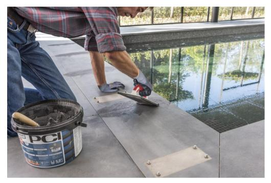
PCI Nanofug Premium was used for grouting the fully vitrified tiles on the pool surround.
