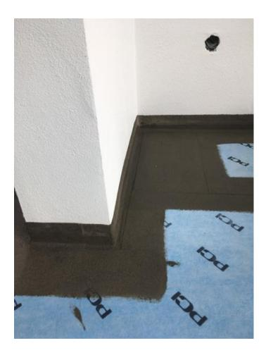
The overlaps of Pecilastic W and PCI Pecitape 120 were bonded using PCI Seccoral 2K Rapid.
