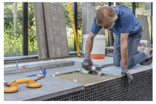
Fliesen-Engelke GmbH used PCI Flexmörtel S1 Flott as the adhesive for the 90 x 90 centimeter fully vitrified tiles. This flexible tile adhesive combines extremely convenient use with a long working time and fast setting.
