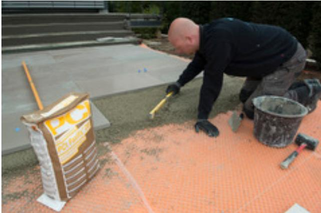
Accuracy comes first: once a 5 cm thick layer of PCI Pavifix DM has been applied, Benjamin Wyß checks the evenness of the surface.
