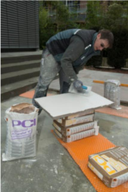
Step by step, the patio takes shape. In order to ensure optimum adhesion, the tilers apply CarrafloTT NT to the back of the natural stone with 6 mm toothed trowel. The slab is then turned over and tapped into place in the fresh Pavifix DM mono grain screed.
