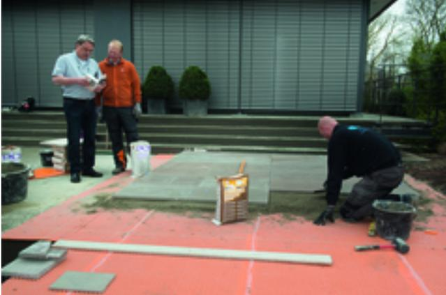
A Schlüter single grain mortar membrane is laid before a 5 cm layer of PCI Pavifix DM drain and screed mortar is applied.
