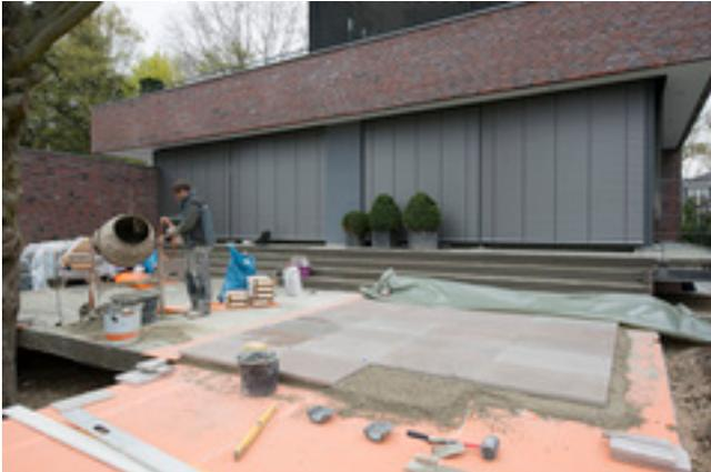
The Pavifix DM is mixed with water in a free-fall mixer before being applied to the single grain mortar membrane in a 5 cm thick layer.
