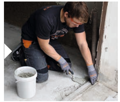
Alternatively filling with mortar
