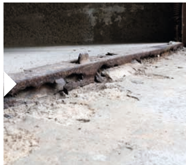
Adjusting the height offset at the entrance rail with a ramp
