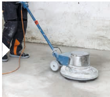
Grinding the floor
