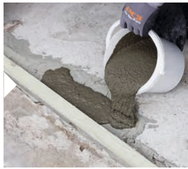
Backfilling the driveway rail with flowable mortar
